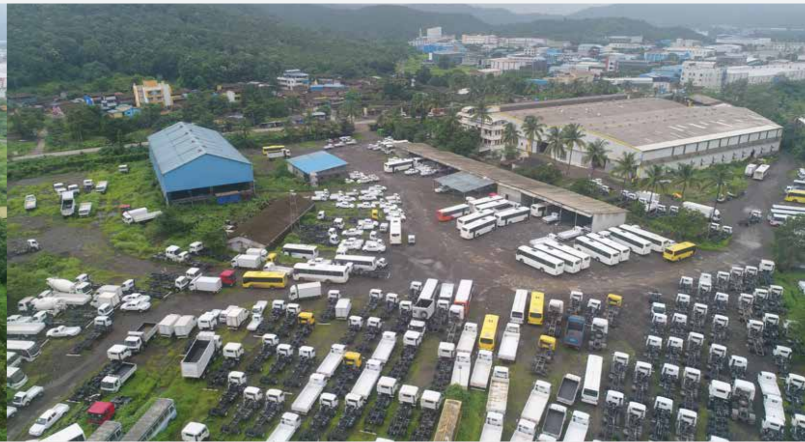
Factory at Patalganga, Maharashtra
